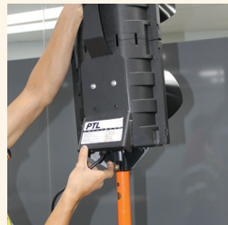
Step 9: To fit the lights, pull spring pin and lower onto post. Release the pin into the fixing hole.
